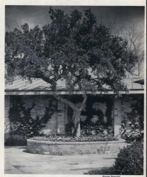
Lowering the soil level around a tree can be disastrous unless a raised bed is built around it before the regrading is done. This one is of brick, with drainage holes at the bottom, and is planted with ivy as a ground cover.
