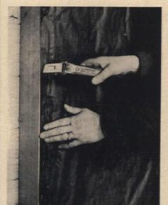
can be insulated with blanket insulation which is placed between wall studding and fastened in place with staples or large-headed roofing nails. The nails are driven through flange on edge of insulation vapor barrier. Flange should be flush against edge of insulation and care should be taken not to tear vapor barrier
