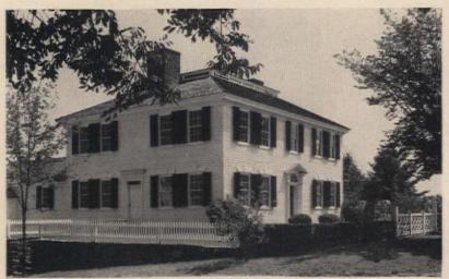
OMINATING the Green at Old Sturbridge Village is the Salem Towne House, built in 1796. Its hip roof is marked by a so-called monitor top roof, with a string of small windows to light the attic.
