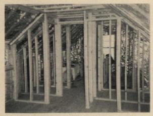
FIRST STAGE of remodeling reveals partition framing and foil-backed insulation in place. View from bedroom shows edge of storage unit at left, under roof eaves. Gypsum board is installed next, right over framing.
