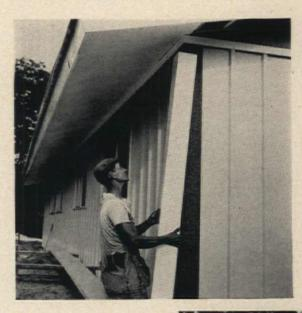
wall and roof panels are erected over concrete slab at building site. Above, workman installs aluminum corner molding after aluminum-covered wall panels are all in place. At right, 4x18' roof panels are laid over aluminum rivet strips which are attached to purlins that lie at right angles to wood roof trusses. Fascia at eaves' edge is also aluminum.
