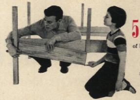
wood PIECE framing metal mesh on side of bed has been grooved to hold mesh. At this point, fasten wood rim in place; glue and screw to the outside of the rail.
