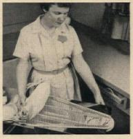
IRONING-TABLE COVER spreads its wings along with the table; need not be removed to adjust width.
