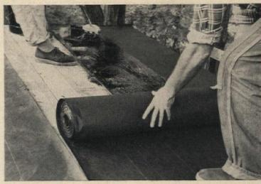
AFTER FIRST TWO LAYERS of asphalt felt are in place along eaves edge, 36"-wide sheets are nailed or stapled to roof deck. Each 36"-wide sheet overlaps the preceding course by 19".
