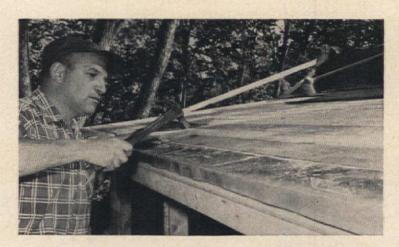
FOR EFFICIENT SHEDDING of water at the roof's edges, install a metal drip edge along the eaves and along rakes. The metal sheeting should be resistant to corrosion and extend 3" back from edge of roof. Bend down over roof edge.
