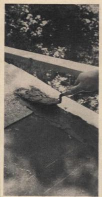
AT THE RAKE EAVES, cement each shingle with asphalt cement to the metal drip edge and to the shingle below it.
