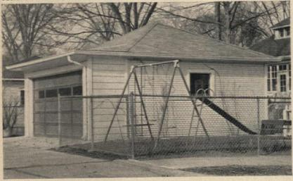
FRONT END of garage was lengthened here because of property line behind garage. Notice how well roof of addition blends in with roof material and lines of the original.
