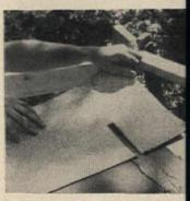
FIRST COURSE OF SHINGLE installed at the edge of the roo is turned to face up the roof
