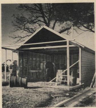
IF YOU EXTEND the rear of your garage, you don't have to move the door. Frame the walls with 2x3 or 2x4 studs; double 2x4 headers over doors. 2x4's can also be used for short rafters.
