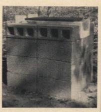
Line fire trough completely with bricks. No part of concrete blocks should be exposed to direct heat. It takes 12 fire bricks to cover bottom of trough. Start at front edge and lay three bricks lengthwise along left side, then stand fourth brick upright as a finishing post. Standing brick on other side, with a brick laid flat between, covers back edge. Put one brick crosswise at front edge. Remaining five bricks fit in with three laid crosswise, two lengthwise.
