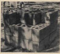
Crisscross the blocks (above) to overlap joints. Top layer (below) is four 6" blocks, two laid flat on each side. So fire trough is 14" wide before lining is added. Lining makes size right.
