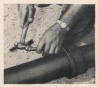
'Only cast iron is really root proof. Joints are packed with oakum and sealed with molten lead. That seals out roots for the life of the building. Remember: CAST IRON IS FOR KEEPS."
