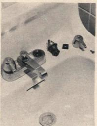
Problem: Leaking fancets waste a great amount of water. Solution: Simply remove the small screw from the handle
