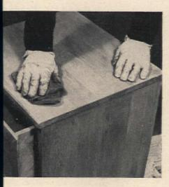
ub dried shellacked surface lightly with very steel wool. Wipe rubbed surface clean with a dry cloth. Repeat steps 8 and 9 two or three e times to build up a hard, durable surface. When you're going to stain unfinished wood, you want it to look like fine furniture. So you go to a paint store and ask for stain. "What kind?" the salesman asks.
