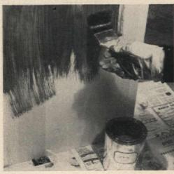
4. Allow "sealed" surface to dry 48 hours. Then brush on ready-mixed stain, quite heavily, following the grain of the wood. To prevent streaking, do steps 4 and 5 on only one section at a time.
