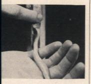
nen you're replacing a broken ndow pane you can apply the tty more easily if you first roll into a few pencil-size strips.
