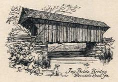
The primary reason for a bridge being covered was to strengthen structure, and at same time to allow interior wood to season.
