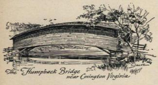
Notice the similarity in roof design between the modern bridge house at right and The Humpback Bridge near Covington, Virginia. Many of the construction ideas developed in our covered bridges are used today. The farther north the bridge, the steeper the roof to shed the snows.
