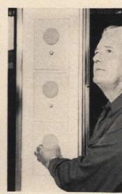
Turn lights up bright for work; or dim them to get "atmosphere." Rheostat allows you to control brightness for the effect desired.
