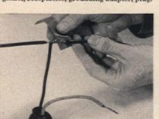
You can make your own Christmas light strings by soldering wires of "pigtail" sockets to bared sections of current-carrying wires. Wrap in rubber tape, friction tape.
