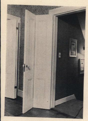
HINGED DOORS solved problem of how to avoid collisions between two doors that swung back against same narrow section of wall. The Harry Curtises of Sea Cliff, N. Y., simply sawed the original doors in half the long way and then fastened them back together with hinges. Now both doors can be swung back against wall with no worries about their banging together.
