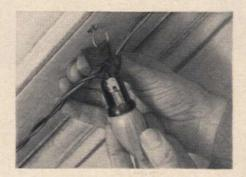
Fasten lamp strings to house exterior with brass cup hooks or insulated staples. Here, lamp string is fastened with friction tape to cup hook that is screwed into roof eave.
