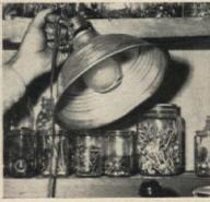
Provide a good, permanent light over each tool in your shop. If a tool is moved to temporary location, it's easy to supply needed light with a simple clip-on fixture. Never undertake even one job without the proper lighting.
