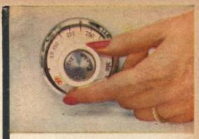
DIAL-TYPE THERMOSTAT regulates "brain." Just set dial at temperature you want. Then the "brain" takes over. Flame goes high when "hot" heat is needed turns itself down to maintain desired temperature.
