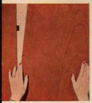
Plankweld's so easy to put up! 16¼" wide by 8' high panels fasten to wall with special metal clips that are then completely concealed by overlapping of the panels. No worry about joints-no nail holes to fill.
