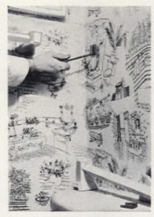
6. To finish off the job, we put up new towel bars and soap dish, then built a frame of furring strips around the tub and basin, covered it with hardboard, enameled the enclosure and all the trim, and cemented the black asphalt cove base to the floor.
