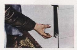
Faster application system saves money Aluminum shadow strip is nailed to studs or sheathing, holds panels in perfect alignment without waves or dips.
