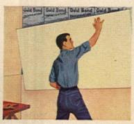
Walls go up fast! Nail big, sturdy panels of fireproof Gold Bond Gypsum Wallboard to the studs. And for a smooth, seamless finish, conceal wallboard joints with the Gold Bond Tape Joint Kit.
