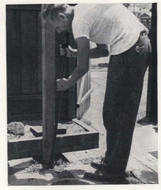
Mix concrete: one part Portland cement, two parts fine sand, and four parts gravel—or use a ready-mixed variety. Pour concrete around each post and work it down thoroughly so that there will be no air pockets. Smooth top of concrete with slight slope for drainage
