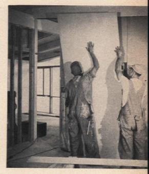
FINAL WALL IS 2<sup>1</sup>/<sub>4</sub>" THICK. Basic panel comprises two Sheetrock panels laminated at mill. On job, a <sup>3</sup>/<sub>8</sub>" thick, <sup>4</sup>' wide panel is applied to both sides of wall
