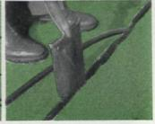
Slit ground 6-8 inches deep with spade. Sink system, heads flush to turf. Tamp.
