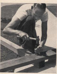
Lay posts on ground, same distance apart as holes. Bolt 2 x 6 beam to post tops, allowing for overhang. To attach to side of house (see
