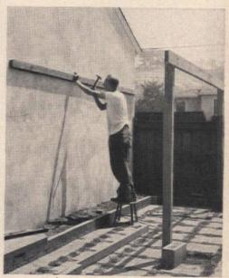
Chock corner posts up plumb. Run a board from top of 2 x 6 to house wall. Level it. Mark wall at bottom of board. Level the notched 2 x 4 beam over this mark, and nail through house siding to studs. One method of locating studs is to tap along the wall—sound is more solid over the studs. A test nail through siding makes sure.
