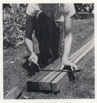
Cut 2 x 4 rafters to extend from wall to 2 x 6 beam. Allow for 2' overhang. Notch one end of each rafter about 1½" to fit 2 x 4 beam. Line up rafters; draw lines across tops about 6" apart, to guide when you nail on top strips
