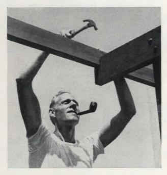
Place a rafter across beams and mark for second notch (to fit 2 x 6 beam) and notch all rafters  $1\frac{1}{2}$ " deep at this point. Fit notched rafters into notches in beams and nail securely to both beams with rustproof nails
