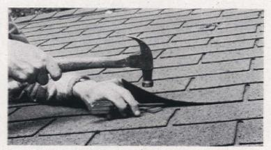
6. If shingle above is too brittle to be lifted without danger of breaking, press nails in with your thumb, then drive them home using a block of wood and a screw driver as shown. Be careful not to hit shingles with hammer. Coat all nail heads with roofing cement
