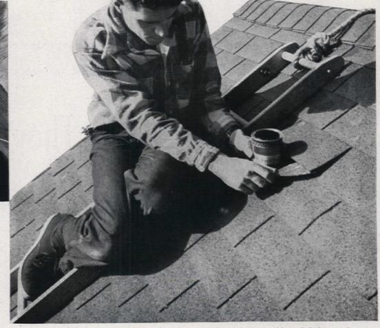
2. Take every feasible safety precaution when you are on the roof. Wear rubber-soled shoes and keep off your feet as much as possible. Don't go up on a wet day—it may be slippery, particularly if your shingles are wood. To use a ladder as a working scaffold, throw a heavy rope over the ridge and pull ladder up, as shown. Tie other end of rope securely to post or tree
