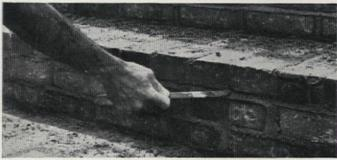
Closure brick (last brick installed) should not be on end of course. Spread mortar on sides of bricks already in place. Set in closure brick without disturbing its neighbors. Tool joints before mortar sets—vertical joints first. Scrape out and compress mortar. (A pipe slightly larger than joint may be substituted for a professional finishing tool.)
