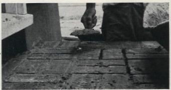
Slush mortar into cracks between bricks, then tool joints. Ten days later, clean bricks with solution of one part muriatic acid, ten parts water. Rinse with water immediately, and thoroughly. Then add hand railings of your choice to finish the job
