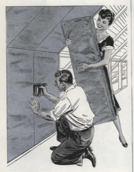
OLD BOND Twinsulation gives you more for Tyour insulation dollar! It provides double insulation action...the rock wool center blocks heat and the aluminum covering reflects heat from both sides. Blankets add extra fire protection...the rock wool center is fireproof and the aluminum covering is flame resistant. The blankets are permanent...their rock wool fibres can't deteriorate.
