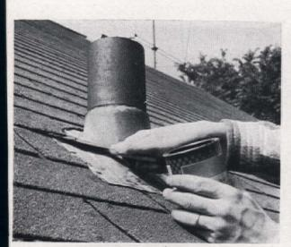
10. Check flashing around plumbing stacks and vents in the same manner as you did around the chimney. Treat by nailing down all raised up lead flashing and by covering joints with a liberal application of roofing cement
