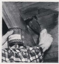
11. In an emergency, it may be possible to repair a leak from the inside. Force roofing cement into leaks or into the cracks between the sheathing boards. Then cover cement with a piece of tar paper cut to size
