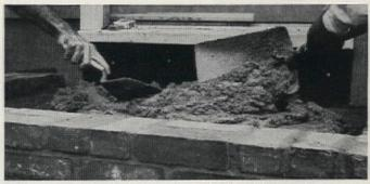
When steps are finished, fill cavity with old bricks or rubble, and cover with kind of concrete mix used for footing. Bring concrete level with top of last course. After concrete sets, apply a level mortar bed. Place bricks on mortar flush with top course
