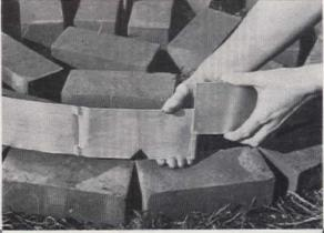
2. Unroll metal strip and place on outer row of brick with notch down and in direction of water supply; lock ends together as shown at left. Next, place circular piece of plastic screening on bricks, with spike protruding through hole in center. Then replace water pipe, passing it through notch, as seen below. Now fit straight ends of curved wire ribs all the way into slots on outside of metal strip until tips rest firmly on the bricks
