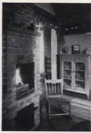
Kitchen fireplace sports a woodbox below, with firebox built at nonstoop level. Brick wall extends to form a convenient work counter
