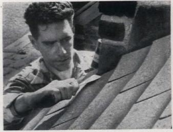
9. Hard-to-locate leaks may often be traced to faulty flashing around the chimney, for water may seep under shingles before dripping down. Check for cracks or holes in flashing. Replace or nail down loose flashing and patch holes and joints with a generous coat of cement
