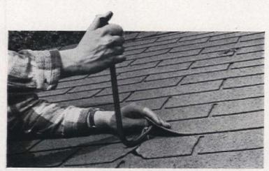
4. If shingles are badly torn or have actually fallen out, you must replace them entirely. Raise the shingle directly above the damaged one and pull out all nails that hold the battered shingle. To remove a wooden shingle, slide hacksaw blade under it to cut off the nails
