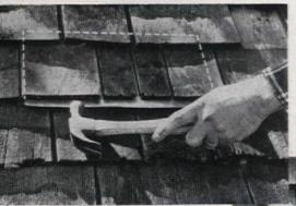
7. If leak results from a split wooden shingle, drive a piece of copper, aluminum, or galvanized flashing under break.
