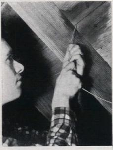
1. To locate leaks in an unfinished attic, look for pinholes of light or for water stains. Slide a wire through hole so you'll be able to spot the leak easily when you're topside. In finished or insulated attics, look for wet spots after rain. Since water may run down rafters before appearing, measure distance from gable and ridge to leak. When you're out on the roof, look all along rafter line above wet spot to find water's point of entry
