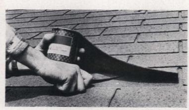
3. If leaks are caused by loose or upturned asphalt shingles, fasten them down with blob of roofing cement placed underneath. Nail down curled edges, and cover nail heads with cement. Repair similar leaks at ridge or hip coverings in the same manner
