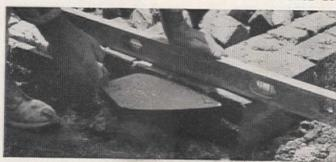
Continue laying courses with bricks at right angles to those below, or lay with overlapping joints. Cut off excess mortar on outside face, flush with course. Watch to see that work is true to plan; use level to check vertical and horizontal accuracy
