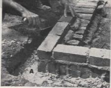
sufficient mortar on end or side of brick to be laid. Do not attempt to lay the bricks and then slush the mortar into the cracks between them, as such joints are not sturdy
