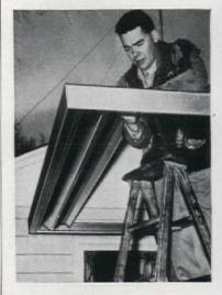
Insert first louver in position and attach to side channels through holes provided. Hole in center of louver should face up. Bolt top channel to louver through center hole, then bolt remaining louvers in place. Louvers alternate to form a pattern of "W M W M W" . . . and overlap to keep out water
