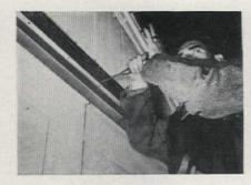
Attach corner clips to 20' channel, and anchor channel securely to building at desired height (we suggest 7'6" from ground). Dig footing holes if required
