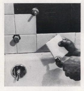
12. Polish tile face with dry cloth. Reinstall tub fittings using pipe joint compound. Wet grouted joints with sponge several times during next four days so grout will "cure" and become waterproof. Seal tub-to-wall joint with caulking
