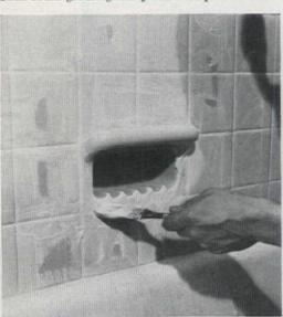
3. Spread adhesive with special notched trowel, depositing on wall only the amount of adhesive that passes through notches when trowel is held firmly against wall. Cover only a few square feet at a time. Do not leave any bare spots
