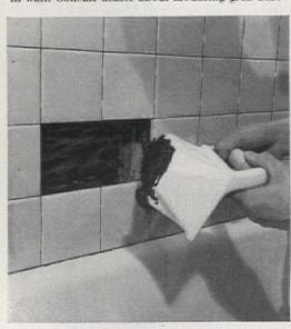
2. Use adhesive to waterproof tub-to-wall joint and around all fixtures. If wall is gypsum board, seal all joints with adhesive. Brush one coat of primer over entire area to be tiled. Give shower area two coats to ensure thorough waterproofing
