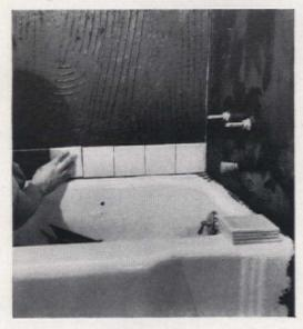
8. To fit around pipes and fixtures, use nippers or pliers to break off small pieces of tile. Take many small "bites" rather than a large one. If the fixture is not on tile edge, cut tile on line centered vertically on fixture. Then take "bites"
