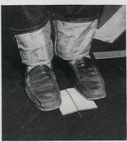
11. Use window squeegee to clean grout from face of tile and force grout between joints. Go over joints with round-ended stick to shape them and force in more grout. After grout reaches initial set, clean tile faces and joints with damp sponge
