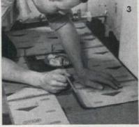
4. Use special trowel to spread the adhesive on floor. Spread it thin; if you use too much it will work up through joints later on. Do a square yard at a time, and plan work so that you won't walk on freshly laid tile
