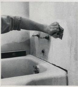
upwards and sidewards. Press tiles on with slight twisting motion. Space lugless tiles 1/32" apart by placing two toothpicks between each tile.
