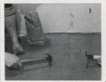
1. Unless floor is level concrete or a double wood floor in good condition, cover it with hardboard underlayment or waterproof plywood. Space special nails six inches apart in both directions. Leave small expansion space between sheets, and all around sides of the room
