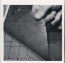
7. Spread more adhesive, and continue laying tile. About an hour after floor is covered, dampen backing paper well and peel it off tiles. If you must walk on tiles, lay a board down first to distribute your weight. Check floor with a straightedge. Realign any tiles that are uneven or high
