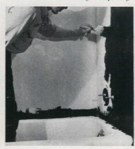
6. To fit second corner, place tile to be cut (A) on last installed tile (B), aligned on edges. Put marking tile (C) over (A) with one side flush against wall and draw line on tile (A). Cut tile on this line to get accurately fitting piece.
