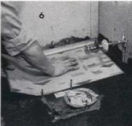
6. Press tiles firmly into adhesive, aligning carefully. Leave space between sheets equal to space between tiles. To cut tiles to fit room edges or around fixtures, use pliers as shown in detail on page 45
