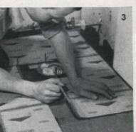
3. To make correct layout, cover floor with sheets of tile, aligning all sheets in their exact final positions. Number sheets on backs. Stack them out of the way and place the first sheets to be used at the top of the pile
