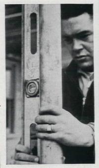
To provide proper drainage, plumb and shim supporting posts so that outer edge of roof is at least one inch lower than inner edge. Bolt pipe flanges to the surface of slab, or fill holes around pipes with concrete to make solid poured footings
