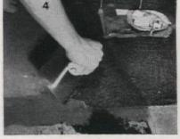
5. If tile coves are to be used at walls, install them first. Butter adhesive on backs of coves. Avoid using too much adhesive. Press coves in place, aligning with straight-edge. If adhesive gets on wall, remove it now with special solvent
