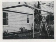
While an assistant holds assembly upright, bolt the two 10' channels to ends of the longer channels to form 10' x 20' rectangle
