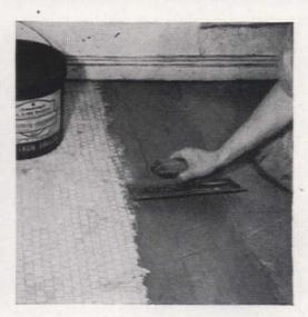
11. Feather out the edges of the filler to make surface perfectly smooth and level. Use filler on any uneven joints between sheets of underlayment or where sheets have not been accurately fitted around edges of the room FOR HOW TO INSTALL LINING FELT, SEE PAGE 92
