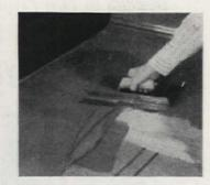
Whether you use underlayment or not, you need lining felt under resilient flooring. First, cover floor with strips cut slightly oversize. Butt joints. Fold each piece to expose one half of floor
