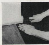
Trim felt around room edges with sharp linoleum knife. Roll edges to get good bond to underlayment. Floor is ready for final covering
