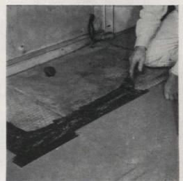
7. Use this quick-fit trick where less than a full sheet is required to fit against wall. Lay sheet to be cut (A) on top of last installed sheet (B). Align edges, As cutting guide, use an additional sheet (C), butted against wall. Scribe B as shown
