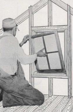
5. Install rough sill at bottom of opening and make it watertight. Put flashing full width of sill, bent down at bottom to overlap siding. At top, flashing starts under siding and comes out to overhang top of trim MORE ON PAGE 86
