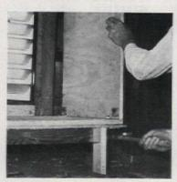
7. In this case, fan crate was used as suction box. Build a sturdy platform for box to sit on, so that it will be centered over louver. A sheet of 3/4-inch insulating board goes under box to reduce sound transmission
