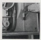
8. Seal space between box and wall with insulating board or canvas and bolt fan in place
