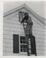
6. Screw louver in place and seal all joints with caulking compound. Cut and fit new trim to match trim of house windows
