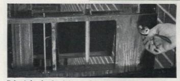
Bolt window bracket fitting to edge of metal window sash after sealing window with weatherstripping provided. Screw intake duct to window bracket, making sure that the whole assembly is centered on window. Test storm dampers for freedom of operation
