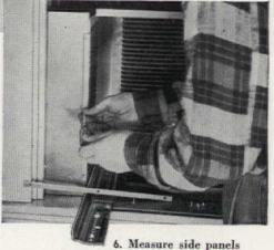
to fit space between outer casing and window channel. Cut panels to size, and slide down into place with smooth surface facing in. Drill necessary holes. Mount securely
