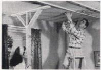
Secondly, apply ingenious Upson Floating Fasteners to furring strips. Then clinch Upson Kuver-Krak Panels into place. Strong-grip Float-ing Fasteners do the rest, hold Panels secure for a lifetime. No visible nailholes, either.
