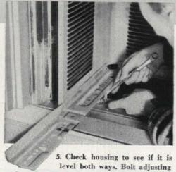
angle to housing and tighten bolts between angles and mounting frame support. Inner sill clamps are provided for some machines
