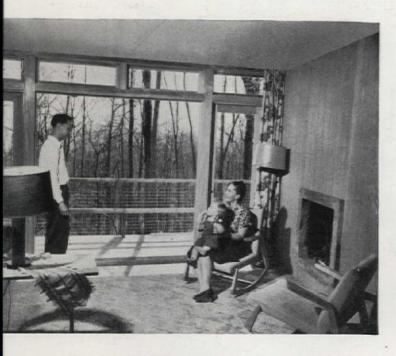
Worth building? This picture tells more than 10,000 words. Fireplace wall was put in at an angle to permit a maximum view of a lake. Concrete and brick fireplace has a circulator that provides adequate heating for a vacation house
