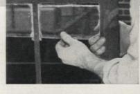
Measure length of window area to be covered by window bracket fitting and cut it to size. Screw fitting to outer storm damper (B)—it goes outside window. Measure sill depth to see if intake duct will extend from fitting to back of machine. If not, have a tinsmith make an extension
