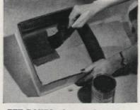
PET BOXES, photographic trays, and waterproof containers can be made from corrugated cartons. Flow liquid on with a brush, allow one hour between separate coats
