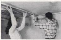
First, right over the present cracked plaster ceiling, you nail up thin strips of wood, called furring strips, sixteen inches apart.
