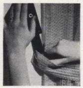
Tie-backs can be stapled to window frames; stapler can pleat plastic curtains for inexpensive window treatments
