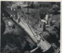
On the floor were built walls of cinder block faced on the inside with ceramic tile, 432 "seconds" costing \$54 plus \$10 for hauling. A regular cement-sand-lime mortar was used, all vertical joints were staggered, and the blocks were interlocked quoin-fashion at the corners
