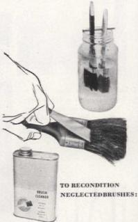
Some brushes can be salvaged by soaking in turpentine or cleaner for a day or two, and occasionally working bristles to loosen old paint. A putty knife or wire brush helps get out dried paint
