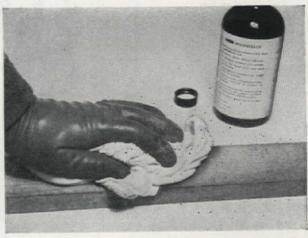
Remove stains and discolorations with a good commercial woodbleach (available at hardware and paint stores). Rubber gloves are necessary to protect your hands
