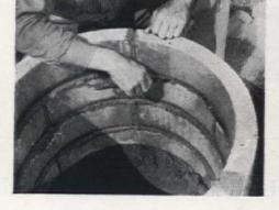
Between third and fourth row, set in steel bars, as shown. They support grill. Decide upon material you will use for fire bed sand is ideal for this purpose. In operation, coals for fire are laid on sand, below grill Leave small drainage holes between sections of first row. Using mortar on top of, and between, each block, build three rows. Keep the blocks level all the way around
