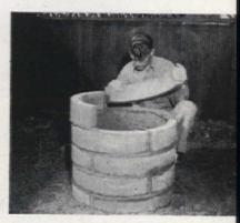
Finally, a half-row, made of two rounded sections, finishes the barbecue proper, acts as a backsplash, and protects the fire within from wayward breezes
