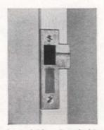
To keep children from locking bedroom, bathroom, or closet doors accidentally, fill bolt hole in plate with putty. For future use of lock, remove putty
