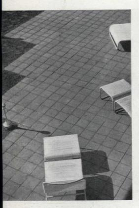
Square paving tile with a slight grout of cement makes an attractive and easyto-care-for terrace. Tiles are laid on leveled area. Provide drainage if needed
