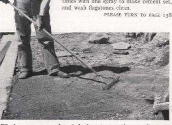
Whether you use a sand or cinder base (a must if you get heavy winter freezing), be sure to grade in a slight pitch for terrace drainage. A rake used upside down makes the job easy
