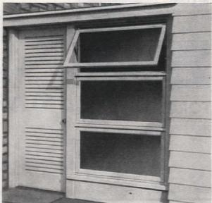
You can have any degree of controlled ventilation with Curtis Convertibles used as awning windows, as here.
