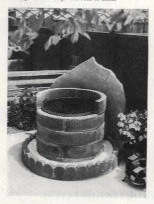
To absorb the drainage, you need a bed of sand, crushed stone, or earth around the base of the barbecue, and such a bed might even be planted. Here the bed is finished off with fluted, rounded curbing. If you can't get it, brick would do nicely.
