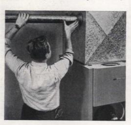
GOT A HOME YOU CAN'T HEAT? No such thing. Even old homes with narrow stud spaces accommodate Blend-Air's versatile new 3½-inch air tubes. They deliver the supply of warm air, or cool air, to Blenders in each room. Pre-engineered and prefabricated to install in a new or old home simply, quickly.
