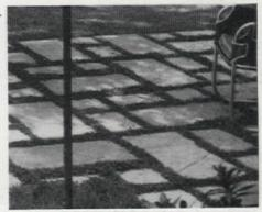
You can pour your own pre-formed concrete paving blocks in wood forms for a barbecue area like this. Plant grass or a sturdy creeper in the dirt between the blocks
