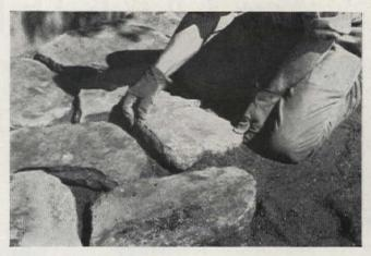
After the base is leveled and pitched, lay down the stones. Fit them together as their shapes permit, but leave a gap of at least a half inch all around each stone. For over-all leveling, place a two-by-four on each end of terrace, and a third board across the other two will indicate any high or low spots. If necessary, work additional sand under stones to make them firm
