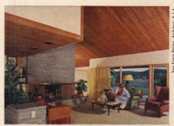
Unusual ceiling is rough sawn Douglas Fir, set on edge and laminated, thus serving as structural material, insulation and interior finish.
