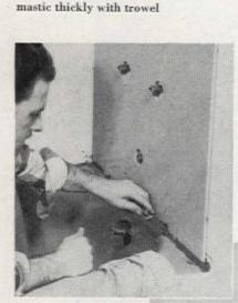
14. Remove excess mastic from rim with putty knife. Set remaining panels
