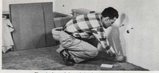
Three simple steps before ordering glass: measure tub wall; measure baseboard; make cardboard templates of plumbing outlets. Dealer supplies mastic and glass cut to size, with holes for fixtures
