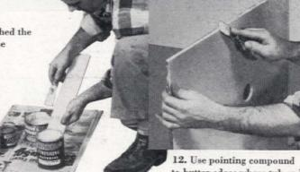
to butter edges where tub end panel butts with back panel
