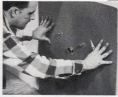
3. For panel under lavatory, make the same type of pattern. With these templates, dealer can cut and drill glass accurately
