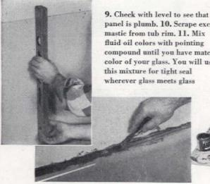
panel is plumb. 10. Scrape excess mastic from tub rim. 11. Mix fluid oil colors with pointing compound until you have matched the color of your glass. You will use this mixture for tight seal wherever glass meets glass
