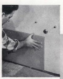
17. Apply base and lavatory panels same way as tub panels. Remember to apply mastic to within 1/2 in. of edges or holes
