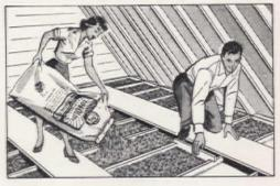
POUR IT, LEVEL IT, LEAVE IT! You'll be amazed how quickly you can do the entire job. Pour ZONOLITE directly from the bag between attic joists and sidewall studs. Flows freely and snugly around pipes, wiring and braces. Just pour and level . . . no muss, no fuss!
