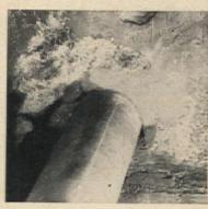
A hole near the sewer line in a basement wall or floor is construed as an invitation by the villain in this tale. All such should be chinked with stones or wire lath and sealed up with impenetrable concrete
