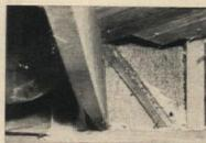
Once rats invade your basement you can expect to see new faces all over the house, for from there they hie themselves into the hollow walls of your house. Spots where walls join the foundation at the sills are especially vulnerable and should be made securely ratproof with metal
