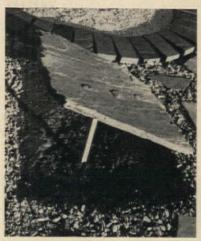
An occasional maintenance job is to fill in under a flagstone that has settled or become unsteady. Simply raise and brace it as shown here, then spread sand beneath it, rake to proper level, and replace stone
