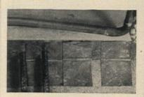
A determined rat finds it no trick at all to slip through even such seemingly impassible avenues as the cracks in old floor boards. In this case "lid" them with strips of metal. Metal is an excellent material for ratproofing in general, and so is cement, since rats can't make headway through either of them
