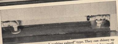
Rats are the "nothing ventured, nothing gained" type. They can shinny up a pipe in nothing flat and squeeze themselves through some mighty small openings at the top. These pipes, uncollared and running to a radiator, invite rat trouble. Once they are fitted with snug metal collars, though, they're proof against the rodents' siege. Remember, even if hole is too small for their bodies, rats can chew through wood PLEASE TURN TO PAGE 154
