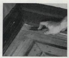
Of course, in the corners an around the radiator, etc., we couldn't use the sanders, but had to go to work with a scraper, steel wool, and sandpaper. Incidentally, whusing the power sander, we swept the floor clean with a brush to remove any solid matter that was not taken up the sander
