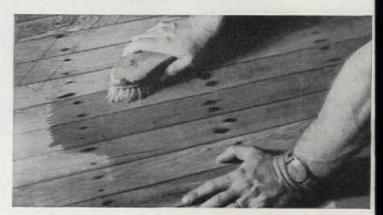
Exposed nailheads had left unsightly black stains on the floor. We had to bleach these out with oxalic acid. We used a mixture of 1 lb, of oxalic acid to each gallon of warm water, and then we applied this to the entire floor with a brush. When the acid was dry, we brushed the floor clean, and rinsed it with three applications of fresh water. After the woodwork dried completely, we gave it another light sanding to remove any of the roughness left by the water
