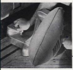
For the edges of the floor, we rented a small sander, called an edger. In this, we used the same grit papers as on the large unit. Edger cost us about \$2 a day
