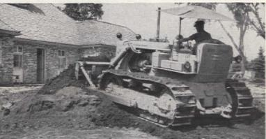
BULLDOZER: If you rent a bulldozer, you can count on its costing from \$6 to \$8 an hour-the fee including the services of an operator. Don't forget that an expertly manned bulldozer can accomplish in one hour the work of two men working two days. In addition to excavating for a house, it's ideally adapted for other large-scale jobs-grade leveling, tree removal, filling in low grade, etc.
