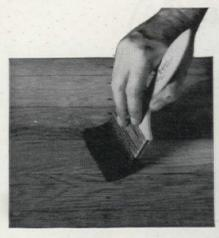
On the bone-dry floor—we waited an extra day to be sure—we applied three coats of shellac, using a 5-lb. cut of white shellac thinned half and half with alcohol. After the last coat had dried (all three can be applied the same day), we sanded the floor lightly with steel wool and dusted it. Then we applied a paste wax. Below you can see the final results
