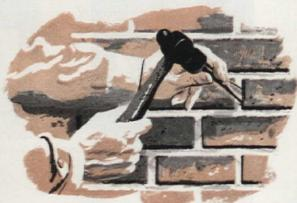
applied over it. Pay special attention to joints between masonry and wood, for in cold weather these open up and allow water to get inside and damage the wood.
