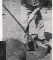
Post holes dug inside metal cylinder did not cave in. As hole deepened, cylinder sank, to be pulled up by its handles when post was set
