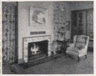
HEATFORM Model "A" for traditional fireplaces. Photo above shows installation with side cool air inlets and, for greater heating efficiency and economy of installation, the front warm air outlet grille. Side warm air outlets may be used if preferred.
