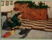
STEP 2... She puts tiles down in place, one at a time. When half the floor is covered, the adhesive is
