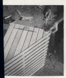
There is only a single row of slats on sides of awning, so nail them closely together. Cut slat tops to follow angle
