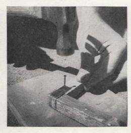
Fasten two triangular frames at top and bottom with strips of 1 x 2 lumber. Add center braces in middle of each triangle and across center front of awning frame
