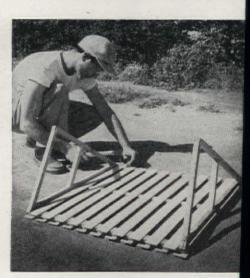
After top row of slats is in place, turn frame over and nail on under row of slats. These should be nailed directly beneath spaces between slats on top row. This will permit leaving top windows open in rain
