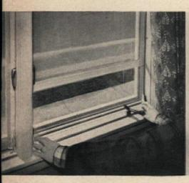
ROLLAWAY SCREENS are installed inside the windows. Press on two small levers and the screens zip up like window shades into a concealed housing at top of frame
