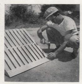
To form a header and add to the appearance of the finished awning, use the long face board which hid the "works" of the Venetian blind. Cut it to fit awning, and nail it in place
