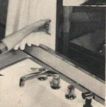
The window remains low, eliminating a costly structural change. It is easily raised or lowered even though it ducks down below the backsplash of the sink, for pulls were cleverly moved from bottom to either side of frame
