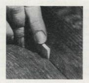
Floor cracks? Clean out, fit wedge of matching wood between boards, glue in, hammer home. When dry, level with chisel, scraper, and sandpaper
