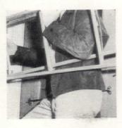
A "buffer" makes storm or screen doors easier to manipulate. Use onepiece towel rod with curved ends. Attach to door hip-high and slanted
