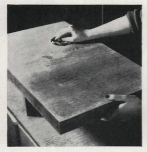
Watch filler carefully. If it becomes too dry, it will be almost impossible to remove. As soon as coat of filler becomes dull, wipe off, against the grain of the wood, with a rough cloth. Rub till every trace disappears and surface is like glass
