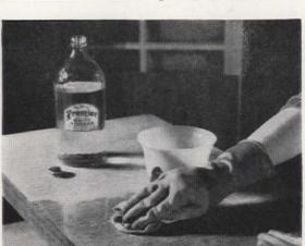
Dry 24 hours, or more if weather is humid. When thoroughly dry, go over entire cabinet with 0000 steel wool to smooth roughness caused by bleach and neutralizer. Surface is now completely cleaned
