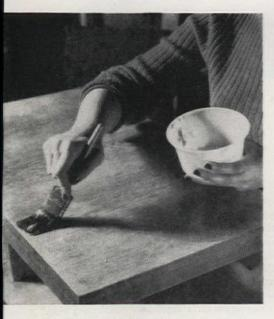
Apply wood filler with an old brush, follow grain of wood. If filler hardens too quickly in bowl, add a little more turpentine. Be sure to cover every inch of surface and put on generously. Do one area at a time
