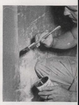
The first coat, with color added, covered the spotted walls completely. A 200-watt work light gave illumination for good vision. A spot missed at this stage would mean a blemish in the strength, texture, and color of the finished enamel surface
