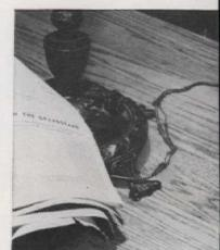
DANGER Such a mass of extension cords may only blow a fuse, but it can also cause the outlet to overheat, fail, and start a fire within the wall where it will get well started before being discovered. For safety, add outlets to your home as you need them. They cost a lot less than a new home
