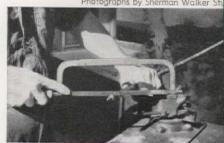
One end of this rod was to be inserted into a wooden wall, the other to be anchored by a screw to a wooden shower frame. After cutting to size, latter end was hammered flat, then screw hole was drilled
