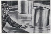
Start of a Long Life! Rheem storage tanks are made by a patent process from steel fused with protective zinc. They're tested under 300 lbs. hydrostatic pressure. And how they last!
