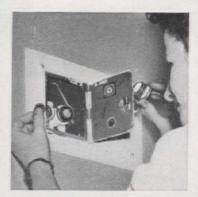
DANGER Replacing a blown fuse with a penny is as good a way as any to burn down the house. Remove the cause of failure, and only use fuses of the right size
