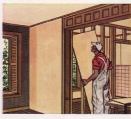
2. Partitions go up fast with fireproof Gold Bond Gypsum Wallboard. It's sturdy as a rock, yet easy to saw and nail. Joints are hidden with Gold Bond Perforated Tape Joint System to make a continuous smooth wall.
