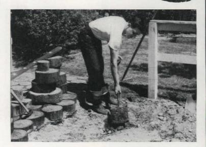
1. Adding to completed portion, collaborator Don Lawrence shows first step, viz., excavating deep enough to provide for a drainage layer of 4 to 6 inches of gravel (more in heavy clay or wet soil) below a 2-inch bed of sand and the log sections
