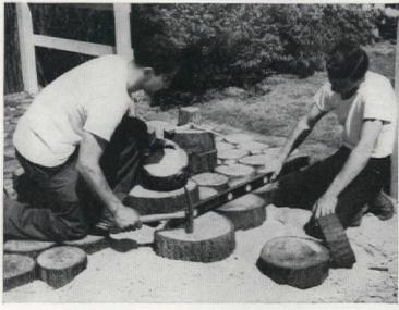
3. Set log sections (as uniformly 5 inches thick as possible) on sand; tap to firm setting with mason's hammer. Take pains to mix different size pieces; see that they touch one another so as to give mutual support and prevent rocking and shifting
