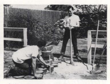
2. After gravel is raked level, tamped firm, spread on it at least 2 inches of clean builder's sand. Rake and tamp this level (as Don is doing). At left, Nicholas Gozo is showing, with ruler, depth of sand layer and of 5-inch log surfacing
