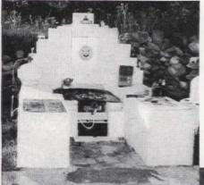
Barbecue pit constructed of cement blocks filled in with dry cinders. 25-lb. drum of butane gas supplies entire season. Gas pressure provided with Reg-O regulation.
