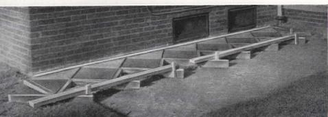
Two sets of forms, as used here, will speed the work. Note the stakes against the long brace, to hold the forms in position. Color may be mixed in the concrete, or sprinkled on the surface and troweled in. Color is obtained from mason's supply companies in powder form
