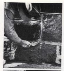
Hold the mortar, on the board, next to the wall and push it into the open wet joints with the small trowel. Pack it tight and add about 1/8 inch more mortar on the surface and smooth it with the trowel. For strong joints and least shrinkage, wet new joints for a few days
