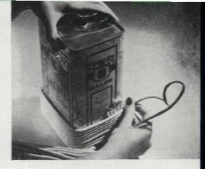
Wrap sash cord round and round oil can. Keep strands close together and very taut. Light fixture attached to threaded pipe that is run through cent of oil can (drawing at right). Paint black, dry, wa
