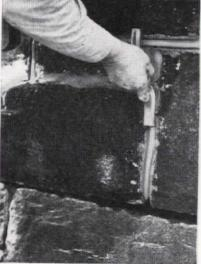
To match a rounded joint in the old mortar, press a round jointing tool in the mortar while it's still soft, and draw it along the joint. This helps pack the mortar, but is mostly for appearance. Scrape excess mortar from the sides of the finished joint with the small trowel
