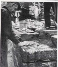
If the cap stone is loose, remove it completely. Clean away all loose mortar and lay the stone again with a new layer of mortar beneath and beside it, after wetting the cap stone and those beneath and beside it.
