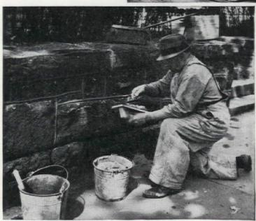
On a mason's hawk, a wood float, or a small board, work a little of the mortar some more with a small pointing trowel before packing it in the joints
