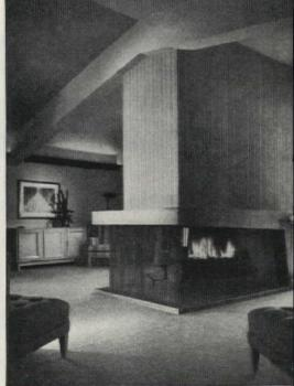
Wide open, this king-sized fireplace throws heat cheer in three directions. Around the tremendous hearth and logs is a metal mesh screen. The roof partly supports the concrete mantel and chimney
