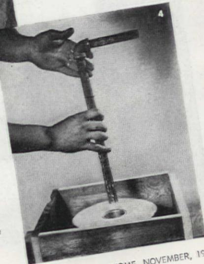
4 Cut piece of 3/8-inch plain plumbing pipe as long as standard for wires and shade is to be, plus depth of base. You also need one elbow and short piece of same pipe for wires at bottom. Put washer on long pipe
