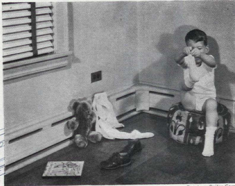
Unobtrusive baseboard convectors spread the heat at floor level along outside walls. This one has fins to heat the air as it passes in bottom and out top
