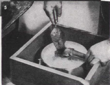
Washer should fit just inside narrow end of cone. Prevents cement from running out. Place pipe through cake pan, elbow at bottom of base. Fill cone with cement
