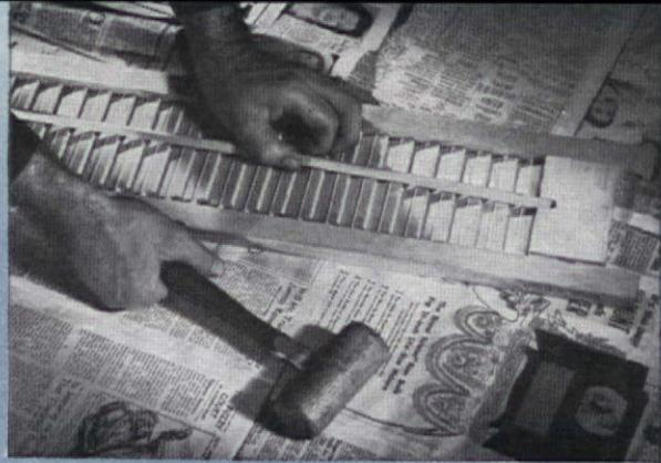
Frame of stiles and rails is assembled loosely, then louvers are fitted in place with a screwdriver or button hook, and the stiles are tapped tightly together
