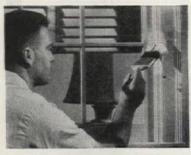
Use the correct brush for each job. Poking large brushes into small corners causes "fingering" of bristles. Cut in around corners with a small brush—one designed for the job.
