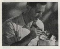
Dip only half the length of bristles in paint—on overhead work dip to only one inch. Tap off excess paint. Don't scrape off on edge of can.
