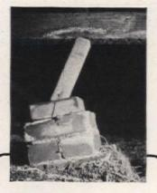
BEWARE! Shallow pier footings will heave from winter frost. Be sure they are below frost line. Hidden plumbing leaks beneath the house (see below) will cause rot in floor timbers as well as provide water for freezing. Look for and repair leaks before more trouble starts
