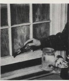
8. Shellac all wooden muntins and sash frames to make good base for paint. Get in corners, so wood will be protected from condensation. Use 2 coats, 24 hours apart
