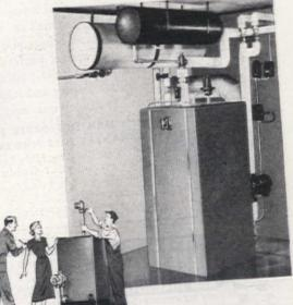
Next comes the B & G Flo-Control 2 Next comes the B & Stightly closed Valve. This valve remains tightly closed except when the Booster Pump is running, preventing heat from rising into the radiators. Hence, it protects against an "over-ride" in temperature and also permits summer opera-tion of the Water Heater.
