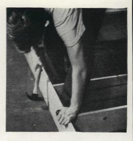
Plain butt joints and good grade of cold glue were used throughout, and sections then nailed together. Top and bottom boards were fastened to sides and then shelves nailed
