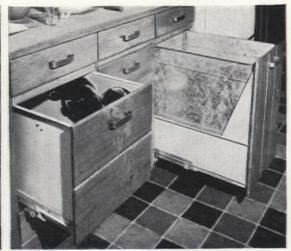
Bottom and center drawers are made of steel, faced with pine. They operate easily on ball bearing tracks like file drawers. Bin holds large wastebasket
