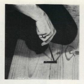
Pieces forming the bottom sections are double-width so boards for lower half were screwed together with iron straps. This saves expense of buying wider lumber
