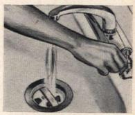
2. Now turn on cold water! This automatically starts action in Disposall hidden below. Food wastes are shredded into tiny bits—flushed away to sewer or septic tank.
