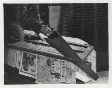
First saw off rabbeted stop on inside edges of old house shutters. Fill all holes with plastic wood. Then, use sandpaper—sand each panel, front and back, smoothly
