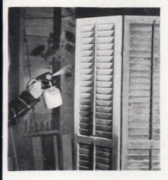
Electric sprayer, or atomizer paint can, makes easy work of painting screen slats. Use lacquer or enamel undercoat for first coat. If you use lacquer, spray several coats. On enamel base, spray enamel. We do not recommend small sprayers for flat paint. Use brush for this
