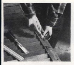
Place one shutter flat on floor. Measure down 8 inches from top, mark with pencil. Then place hinge in position on shutter, as shown. Peneil mark all around hinge. Measure up same distance from bottom. Repeat. Then line up all shutters on floor and mark other 3 to match first shutter
