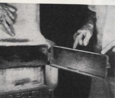
White ash along the center on top edge of this clean-out door and the black area above it are a sign that the door is warped and that heat and coal gas leak into the cellar
