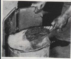
Clean ash, soot and other dirt from the bottom of chimney, through the clean-out door or the smoke-pipe opening. Use a mirror to check the chimney flue for obstructions that must be removed
