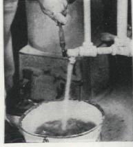
Drain sediment from bottom of the boiler until clean water appears. Then, with a hot-water boiler, refill the boiler and radiators completely, eliminating all air in the system
