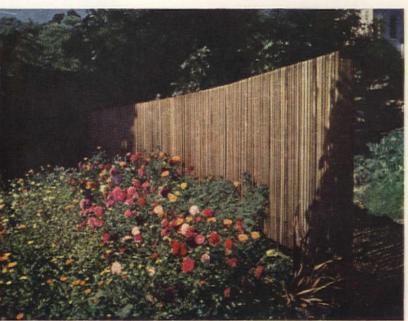
Twelve feet back of retaining wall, a 6-foot fence of  $1 \times 1$ -inch redwood stakes on a  $2 \times 4$ -inch framework provides privacy, background for asters and marigolds (in front) and rampant geraniums partly shaded by walnut tree (in rear). Beyond the fence are the clothes-drying yard and a vegetable garden
