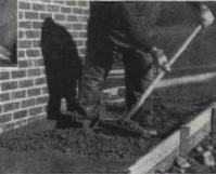
Spread each batch quickly, using hoe or iron rake to get even, solid distribution
