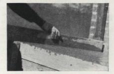
Give desired final finish with wooden float (shown), smoothing trowel, or both. Edge and score with edger
