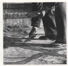
An inexpensive walk, flexible and presenting no frost problem. It is of salvaged asphaltbrick laid directly on well-drained, firmly tamped earth. Hot tar is poured into joints
