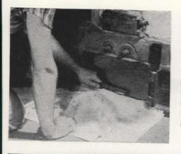
Remove all ash and soot that has fallen to ash pit. Inside of firebox and heating galleries can now be checked for cracks that need repair by welding or with fire clay or iron cement
