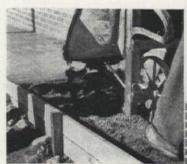
Concrete for making a walk is easily mixed in, then poured from a wheelbarrow
