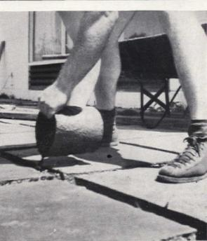
Topping is applied right after 16 squares have been floatfinished. A tablespoon of the dry color is sprinkled on each square and troweled into the topping. Use more color for deeper tints. Concrete is then left overnight for initial set
