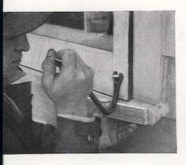
Remove stuck storm sash with a jimmy bar or a claw hammer and eyelets or lag screws in corners of sash. Work corners alternately and gradually to prevent twisting and breaking of glass
