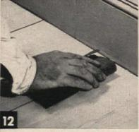
(12) Go over edges of floor with fine sandpaper on wood block to make main area and edge match. Edger cuts across grain at board ends, making texture different from adjacent areas where sanding is with grain
