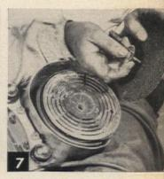
(6, 7) Don't do this! It's expensive at 50¢ a sheet. The paper wasn't tight and even on drum (6), or a nail wasn't set. With main part of floor rough sanded, put a disc of coarse paper on edger (7), to clean room borders. If you can't get round paper, cut circles from large sheets and punch a hole in the center
