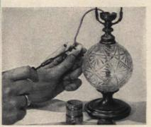
Remove lamp cord from socket by loosening the two terminal screws with small, finebladed screwdriver
