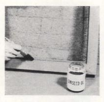
Give all raw wood in rabbet a coat of paint or linseed oil. This prevents excessive drying and weakening of putty or glazing compound from oil being absorbed by wood
