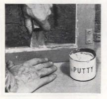
When paint or oil is dry, apply a bed of putty or glazing compound to back of rabbet against which glass will lie and make air- and weather-tight seal
