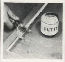
Next apply the putty or compound to junction of the glass and sash frame. Press it in firmly, filling all voids, and being sure to cover glazier's points
