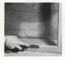
First remove all broken glass. Then clean all old putty from the rabbet, using a chisel and being careful not to gouge the edges in the process
