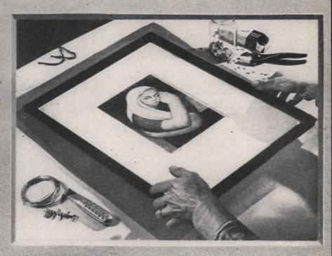
Glazier's tacks or small brads fasten print and glass to inside frame. Cover back edges of frame with glue, lay framed picture face up, on sheet of wrapping paper. Seal paper and edges of frame to make dust-tight cover. Wire and hang
