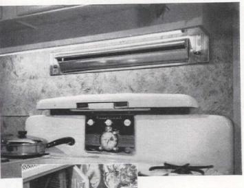
Range-length ventilator eliminates odors, greaseladen vapors and helps keep walls, ceiling, and fixtures clean and bright Garbage container with
