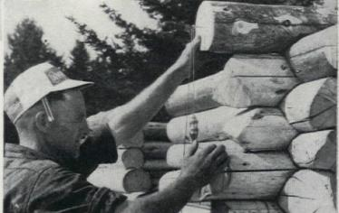
The rough-notched log is laid in place and lined up plumb before marking for the finished cut
