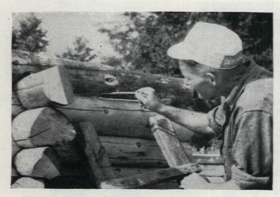
Crayon is used for marking the log after it is lined up. Pencil is useless on the smooth surface
