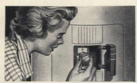
This is the "brain" of the Rheem gas models. The dependable Grayson Unitrol. You set the thermostat for the water temperature you want. The control automatically feeds gas as required to maintain the preset temperature. Goes on and off by itself. Even shuts off all fuel if the pilot light should go out.
