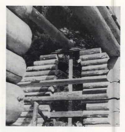
Spikes and props steady and support the gable-end and ridge logs until the chimney is completed
