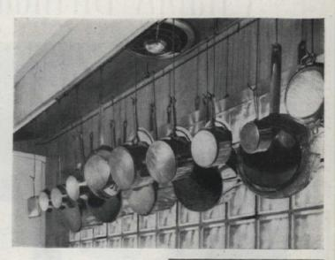
Hexagonal brass rods of varying length with rings at top and hooks at bottom, slide across the steel bar which extends from wall to wall. Cutaway of bar shows storage shelves below
