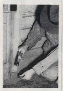
• Rat populations must be eliminated by poisoning, trapping, gassing—then all buildings completely ratproofed. Gnawed edges of wooden doors and sills can be sheathed in metal to prevent new invasions
