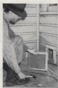
Pieces of hardware cloth, bound in metal (materials available at your local hardware store), will effectively protect ground-level openings. Holes around pipes should be sealed off with cement mortar
