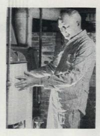
• Furnace insulations can either be trowelled on or applied in sheets that can be wired in place easily
