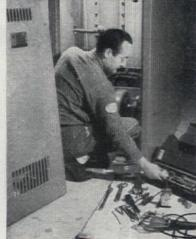
You can remove soot and fly ash with a long-handled brush. Have service man clean and adjust oil burner
