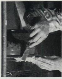
Small leaks in the joints between the furnace sections can be patched readily with asbestos furnace cement
