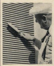
Wire brush is used to scrape off loose paint. Ragged edges and other rough spots are sanded to get surface perfectly smooth. Prime coat is applied to spots where wood shows
