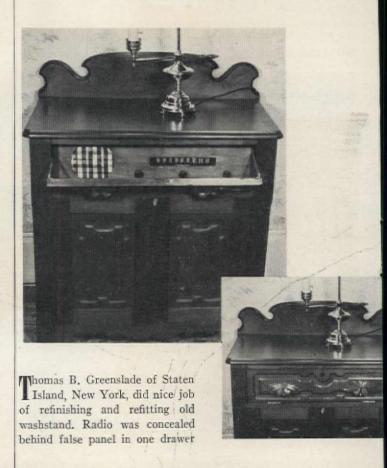
Panel was cut for dial and speaker opening, finished to match repiece. Replaced drawer front drops forward on hinges for access to
