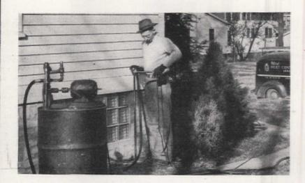
Poison is pumped into soil outside the house at various points. Equipment, besides çod, includes electric pump, hose and hose reel, and oil drum containing poison. For home control methods, see text
