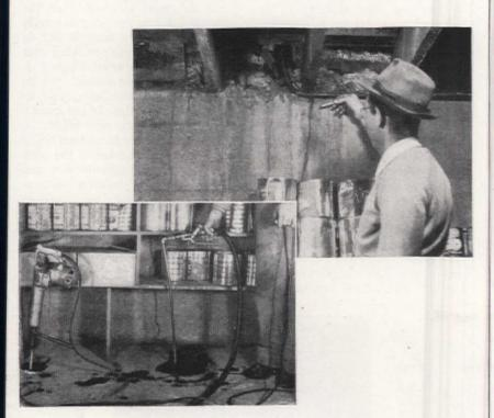
A termite-control man points to a shelter tube that extends up concrete foundation wall to floor of dining room above. When well established in the floor, termites build tubes through a crack down to the earth. Drill is used to bore holes through concrete, then the poison is forced through rod and into soil beneath the floor.
