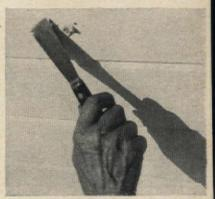
A smoother, better-looking surface results if you putty all nail holes and rough areas around knots. If painting over new wood, touch knots with shellac after the priming coat
