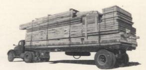
An entire house is delivered. The elements are assembled to be unloaded in sequence
